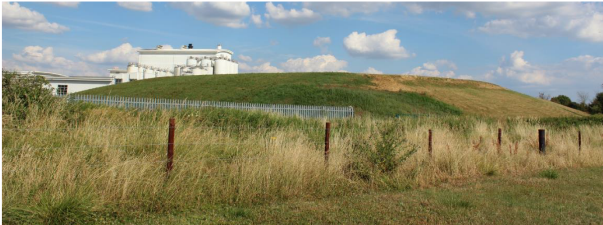
Existing bund beside Arla Dairies site
